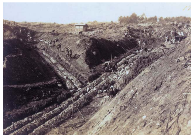
Photo 2-2 Installation of interceptor underdrain at Chausuyama landslide (courtesy of Nagano Prefecture)
