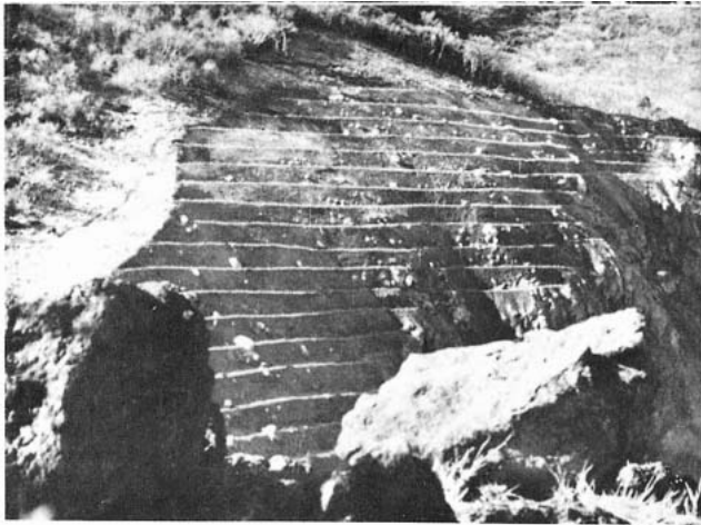
Photo 2-5 Grading work (Earth removal) at Sohunzan landslide (courtesy of Kanagawa Prefecture)
