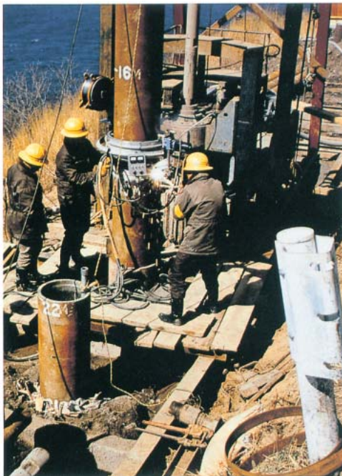
Photo 5-11 Pile driving
