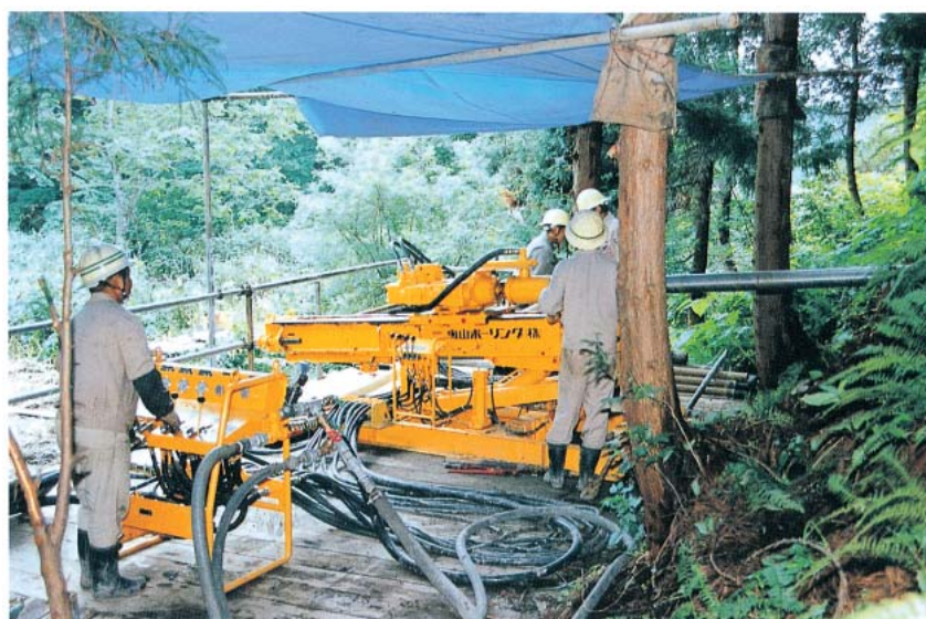
Photo 5-3 Horizontal gravity drains installation
