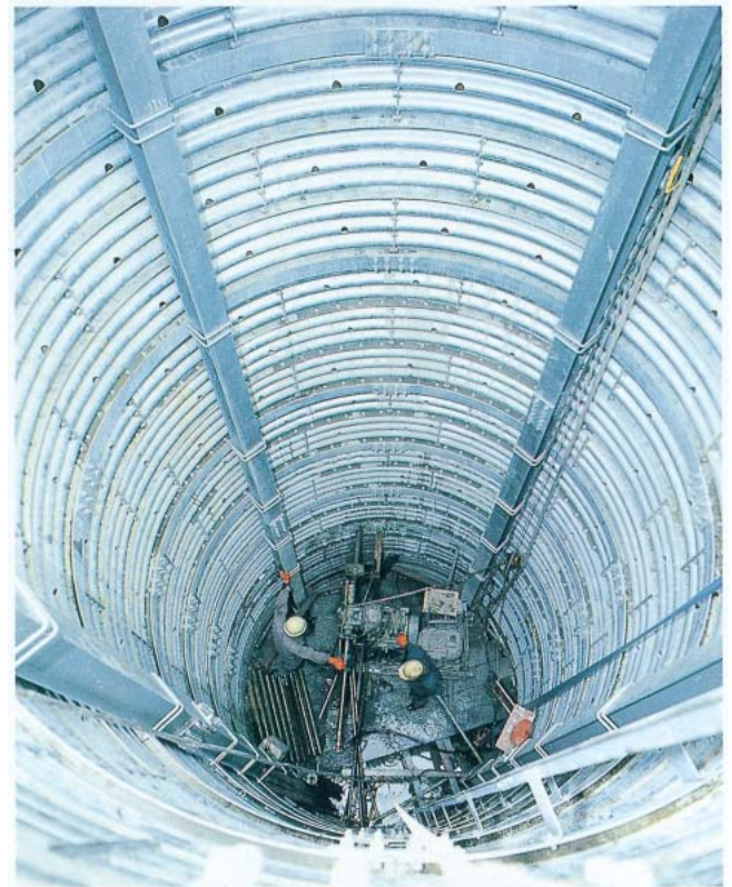
Photo 5-5 Drainage well using steel segments
