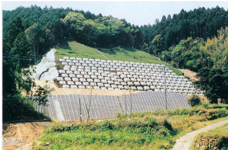
Photo 5-13 Completed anchor installation
