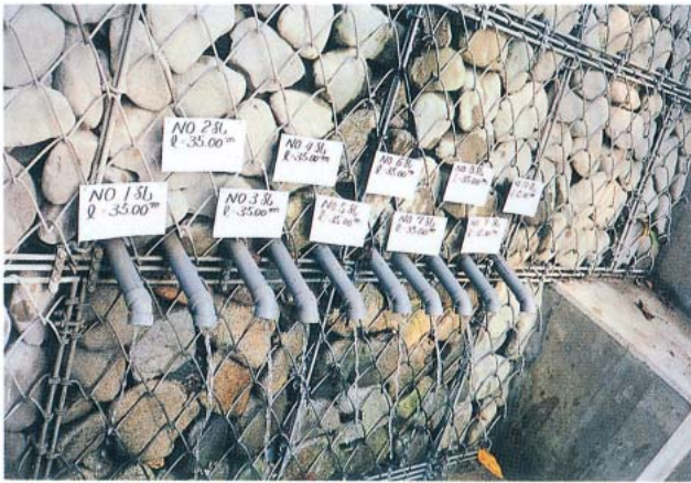
Photo 5-4 Outlet of horizontal gravity drain pipes
