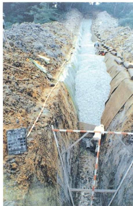
Photo 5-2 Interceptor trench drains
