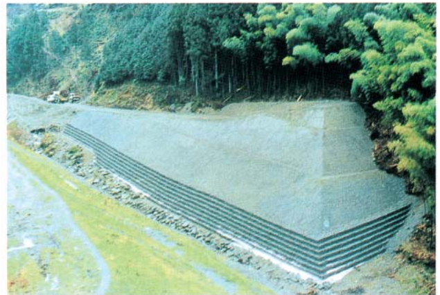
Photo 5-9 Buttress fill
