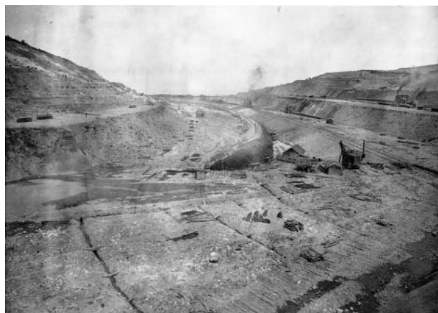
Photo 2-1 Ohkouzu diversion channel (landslide occurred on the right hand side of the photo) (courtesy of Ministry of Land Infrastructure and Transport)
