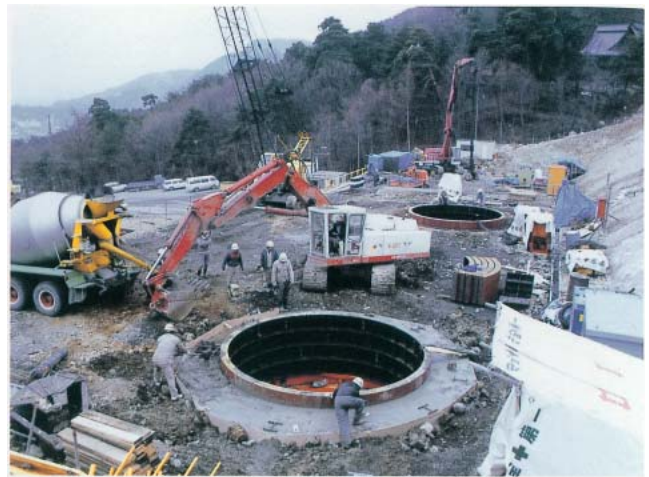
Photo 5-12 Installation of large diameter cast-in-place shafts
