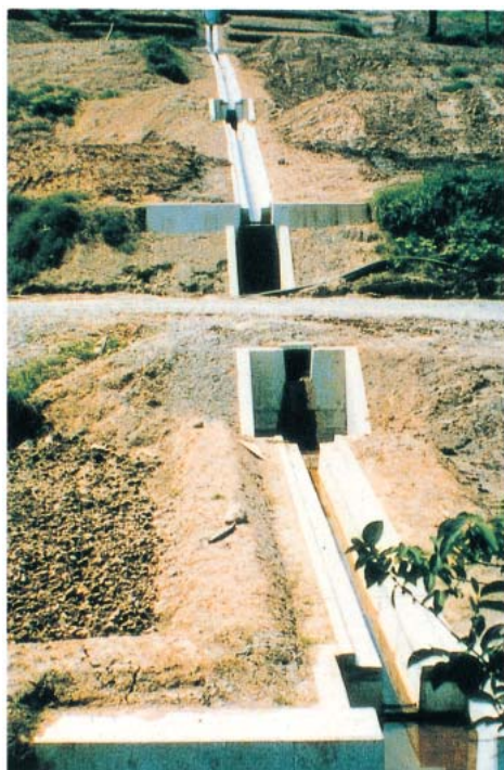
Photo 5-1 Surface drainage ditches
