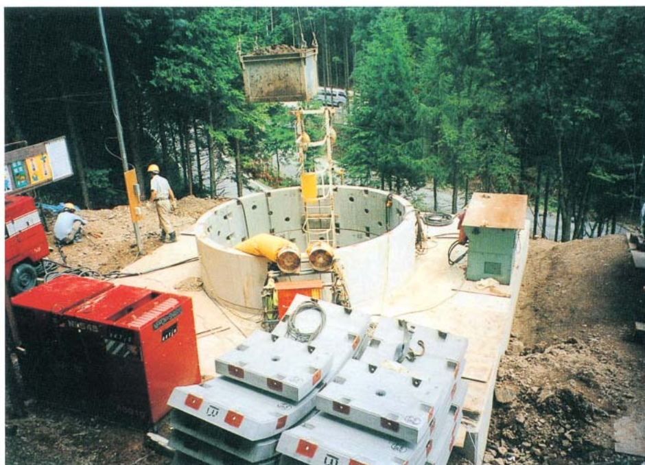
Photo 5-6 Drainage well using reinforced concrete segments
