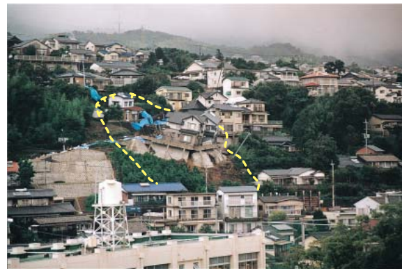
Photo 6-38 Harabun landslide causing damages to residential structures (courtesy of Nagasaki Prefecture)
