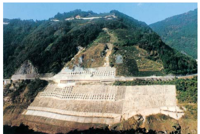
Photo 2-8 landslide at Ohdo reservoir following the completion of anchor installation (courtesy of Ministry of L. I. and T.)
