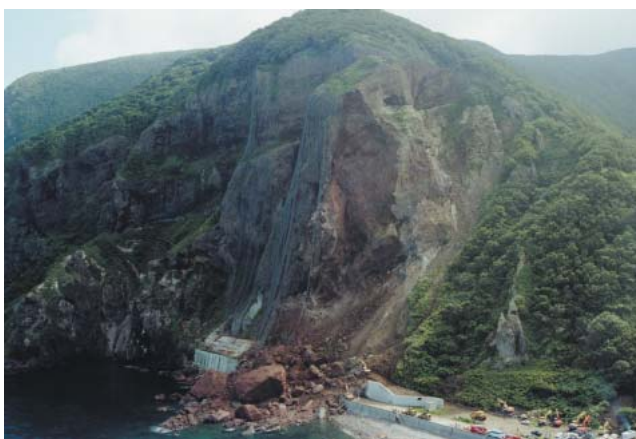
Photo 6-2 Initial fall of rock fall at Daini Shiraito tunnel (courtesy of Ministry of L. I. and T)
