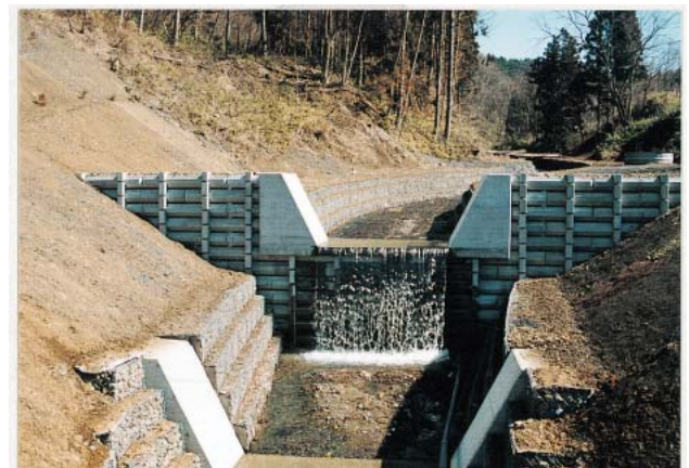
Photo 5-10 Sabo dam (check dam)
