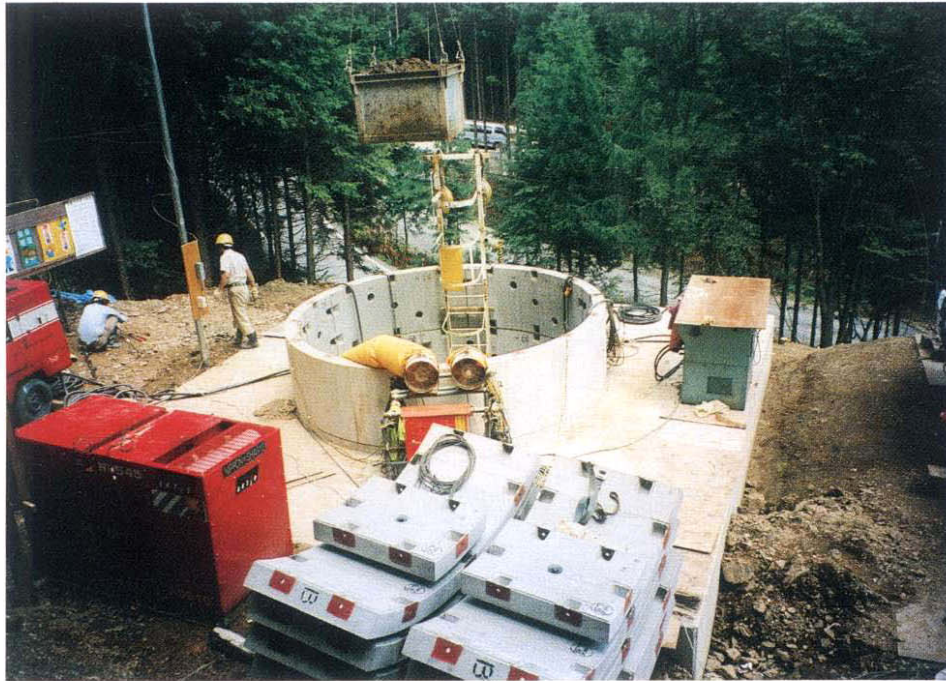
Fig. 42 A drainage well using reinforced concrete segments
