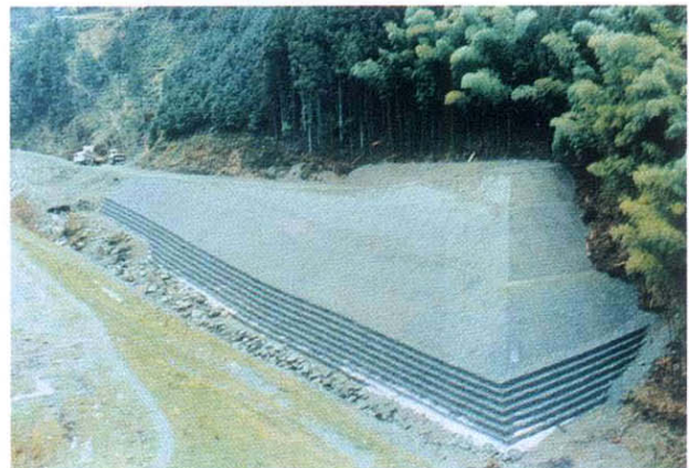
Fig. 47 Buttress fill works
