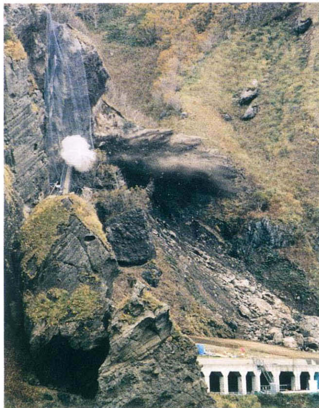
Photo. 2 Blasting of the hanging rock blocks (Photo courtesy of the Hokkaido Shinbun Press)
