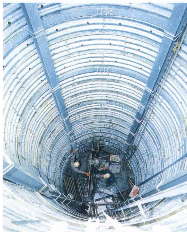
Fig. 41 A drainage well using steel segments
