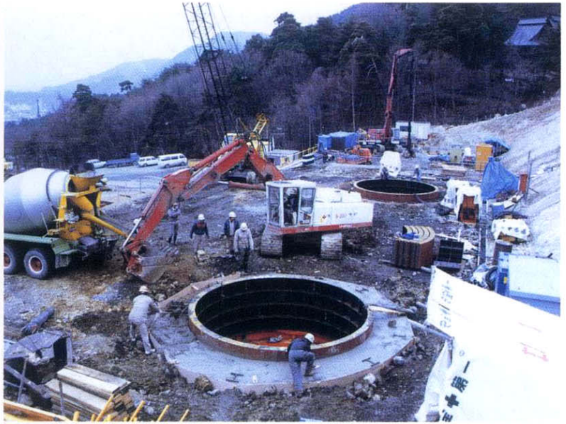
Fig. 49 Under construction of the large diameter cast-in-place pile works
