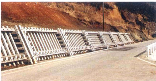
Fig. 51 An example of crib walls
