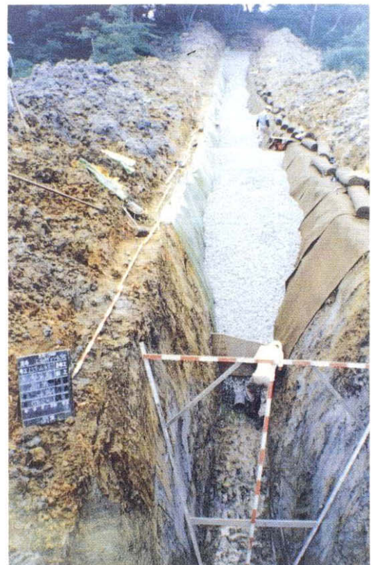
Fig. 38 Interceptor trench drains
