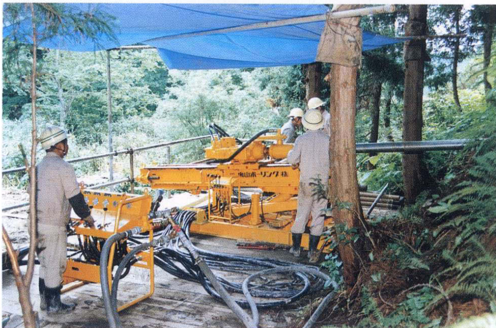
Fig. 39 Drilling works for horizontal gravity drains
