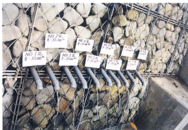
Fig. 40 Outlet of horizontal drain pipes
