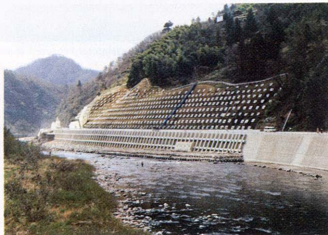
Fig. 5-20 Anchor works to detain a landslide
