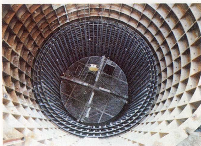
Fig. 5-18 Inside of a shaft using steel segments
