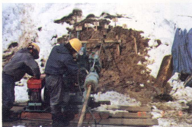
Fig. 5-10 Drilling works for subsurface drain
