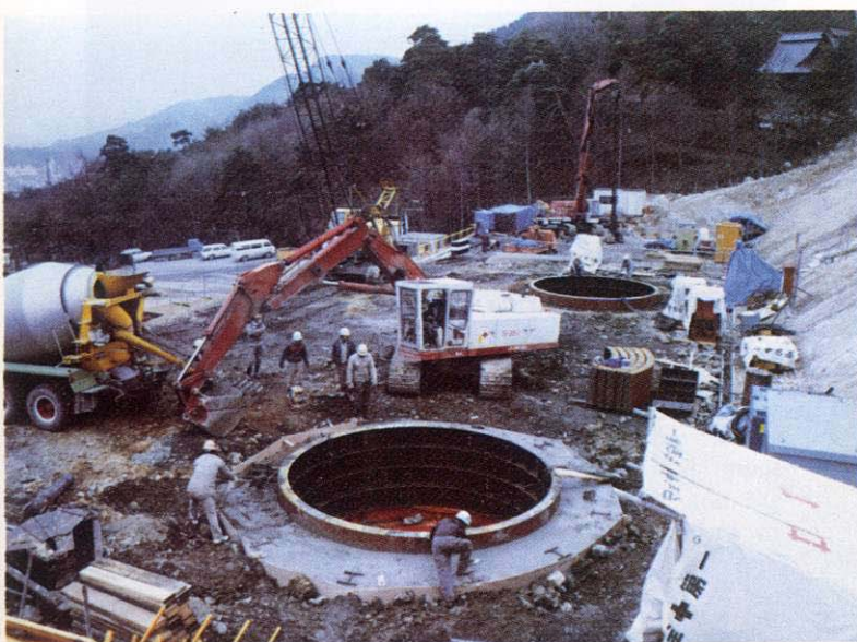
Fig. 5-19 Under construction of the cast-in-place piles
