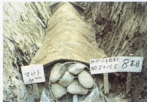
Fig. 5-7 Construction of an interceptor drain
