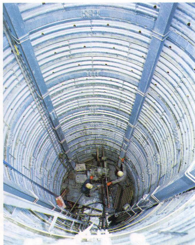
Fig. 5-13 A drainage well using steel materials
