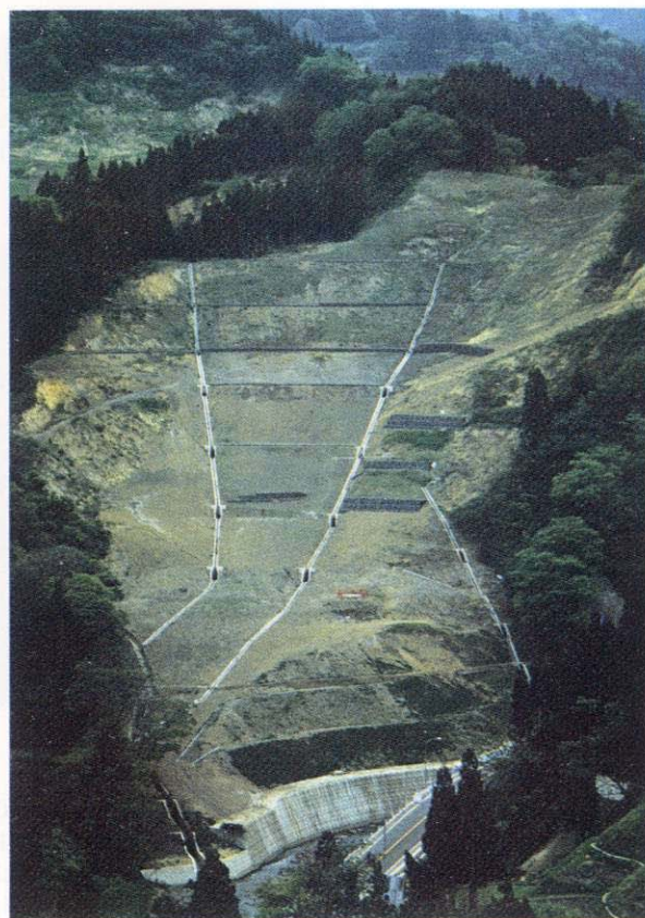
Fig. 5-5 Surface drainage works and soil removal works to reduce the weight of the sliding mass
