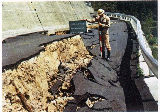
Crack occurrence at landslide head (April 1982)
