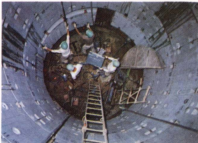
Fig. 5-14 A drainage well using reinforced concrete segments
