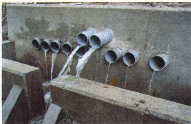
Fig. 5-11 Outlet of horizontal drain pipes
