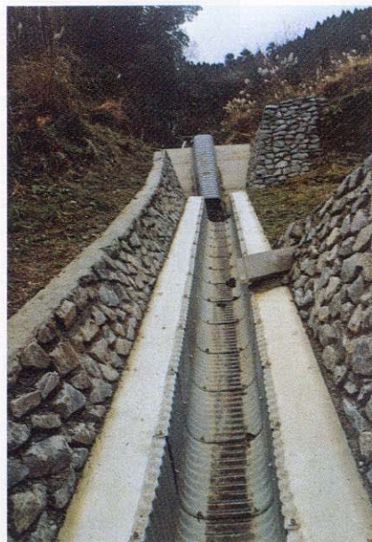
Fig. 5-6 Surface drainage ditches with corrugated half pipes
