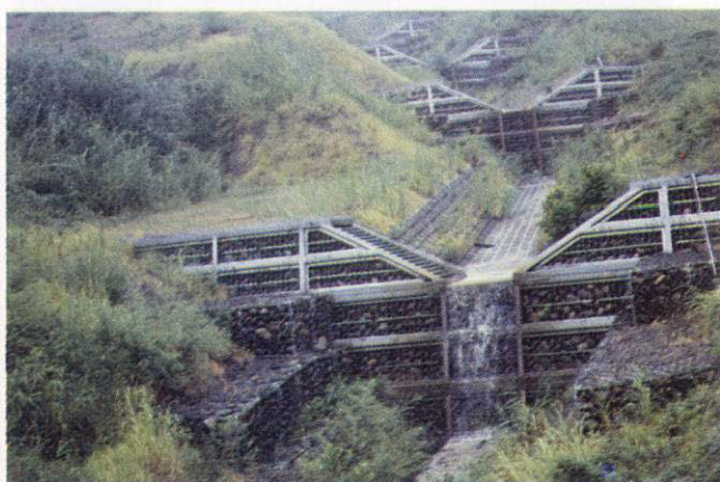
Fig. 5-8 A groundsil using flexible steel frames
