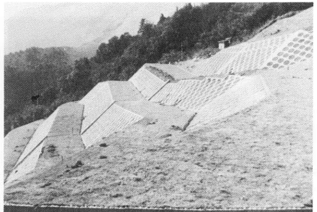
Fig. 6-15. An excavated slope covered with concrete blocks.
