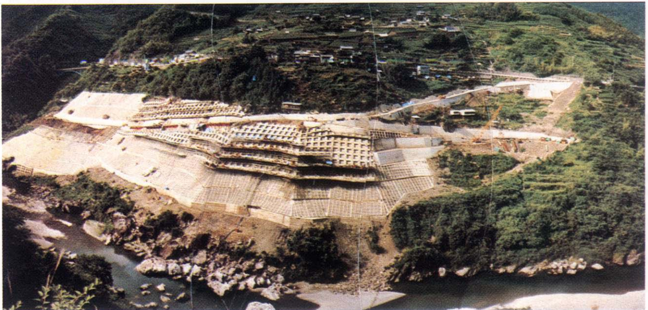
Fig. 6-19. Anchoring for a landslide control. (Odo landslide)
