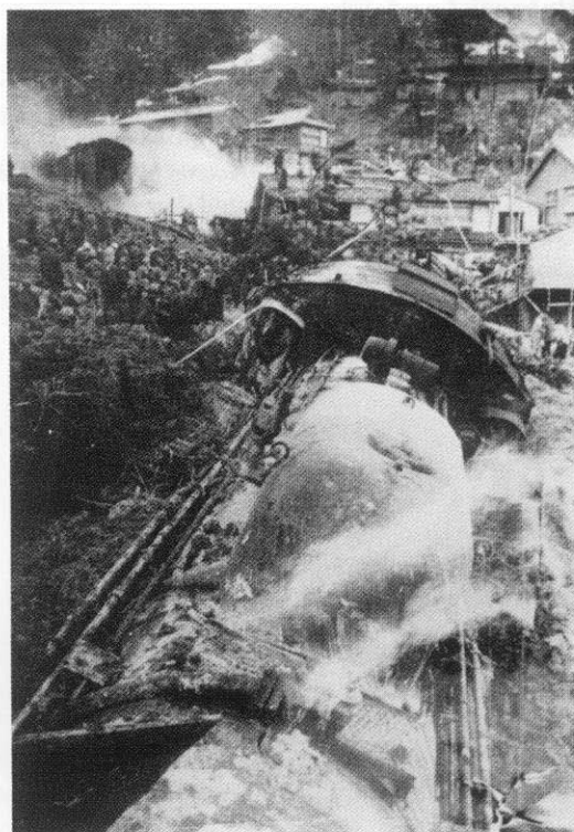
Steam locomotive moved and partially buried by the slid mass (Courtesy of the Niigatanippo).
