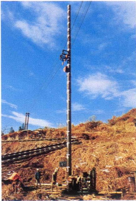
Fig. 6-17. Inserting of a steel pile
