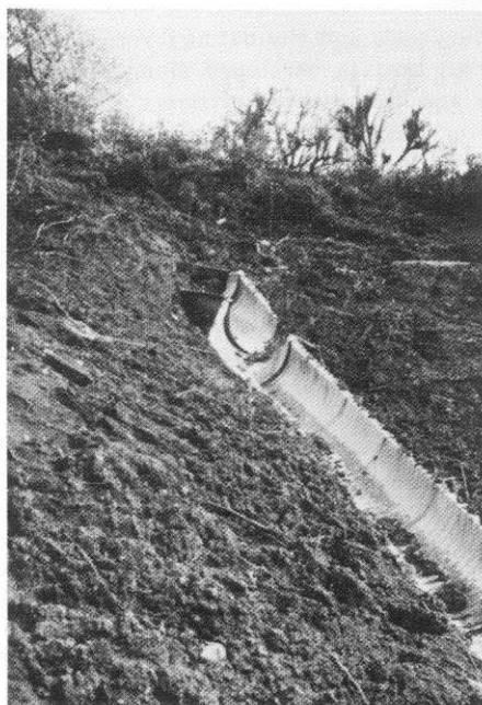
Fig. 6-1. Surface drain of the corrugated pipes.
