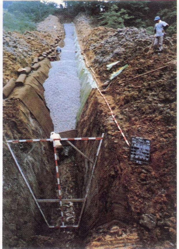
Fig. 6-18. Under construction of an interceptor drain work.
