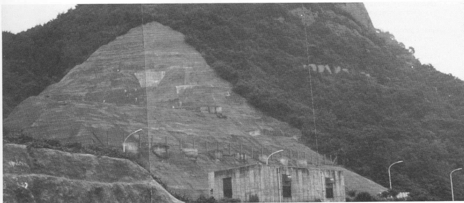
Iwadonoyama landslide after the completion of control works (Photo taken in 1979).
