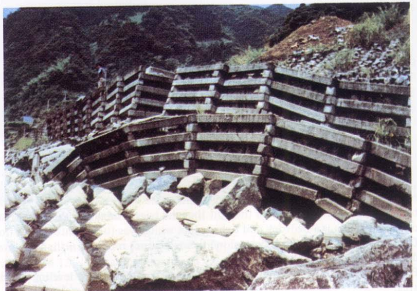
Uplifted crib work at the toe of the landslide (Photo taken in 1979).
