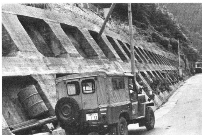
Retaining walls at the lower part of Sakaishi landslide.
