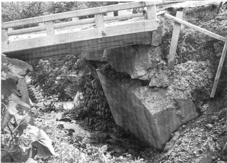
Damage of the Terasawa bridge
