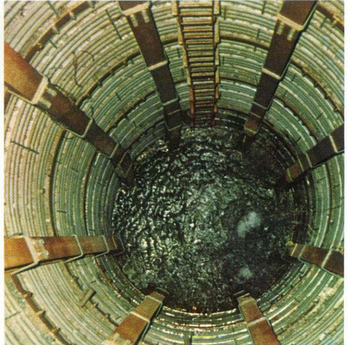
Drainage arrangements and works, a circular structure in the center shows a ferroconcrete well (Chausuyama landslide)
