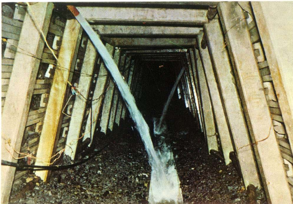
Drainage tunnel, the amount of drainage is about 300 l/min. (Washiodake landslide)
