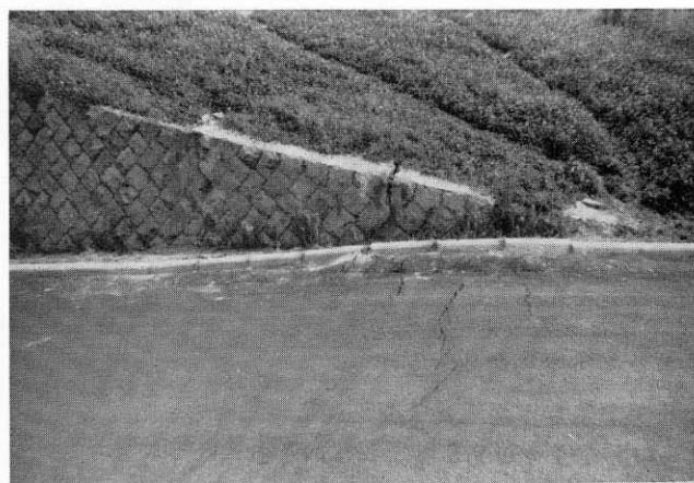
Cracks at retaining wall and pavement of highway.
