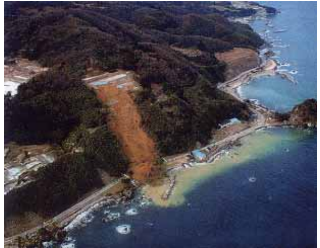
Figure 4. Aerial view of the Katanoo landslide (Courtesy of Kowa Co. Ltd.).
