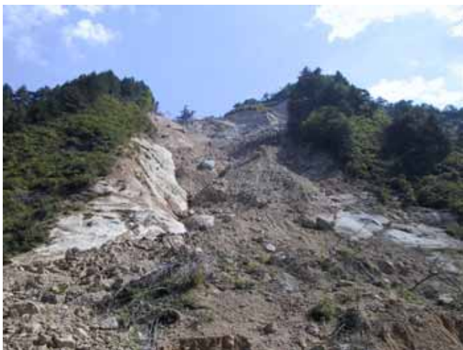
Figure 6. Front view of the Tozawagawa landslide.
