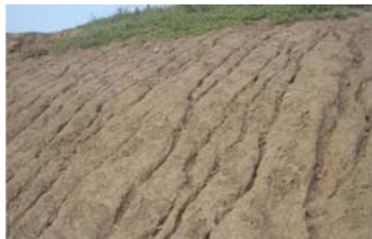
The clayey soil slope of highway in Nanjing, Jiangsu Province, China
