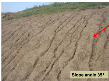
The clayey soil slope of highway in Nanjing, Jiangsu Province, China
