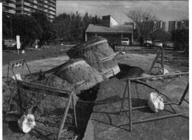
災害用貯水槽が被災
