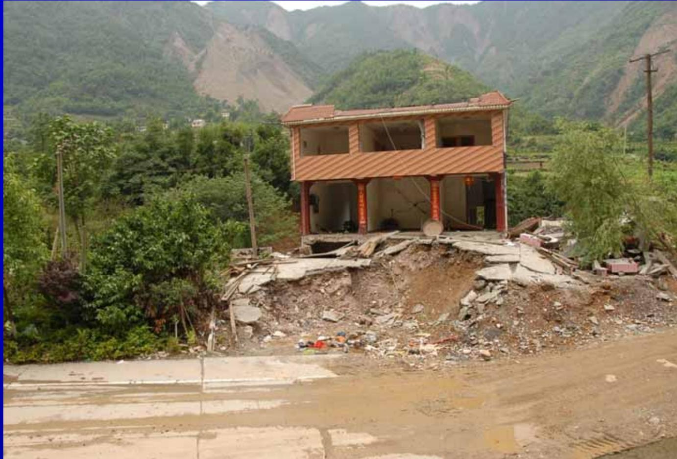
Originally, the house was at the same level as the road. The height of one floor is about 3m, so the uplift of the fault in this position is estimated around 4m.
