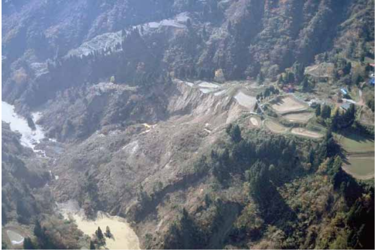
Pic. 5: Landslide at Yamakoshi area due to the Mid-Niigata earthquake 2004
