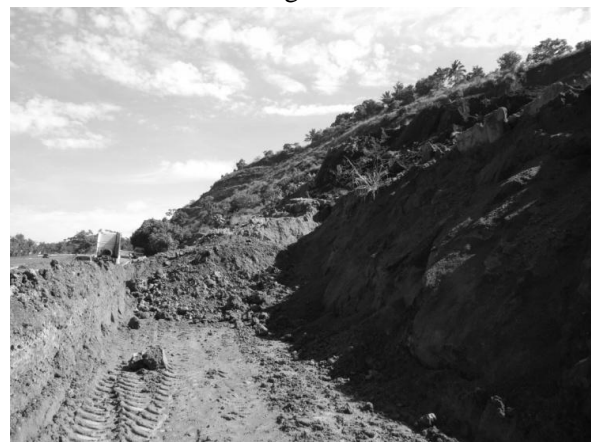
Fig. 37 Toe region of the landslide showing localized surficial failures (Photo taken on September 11, 2012)
