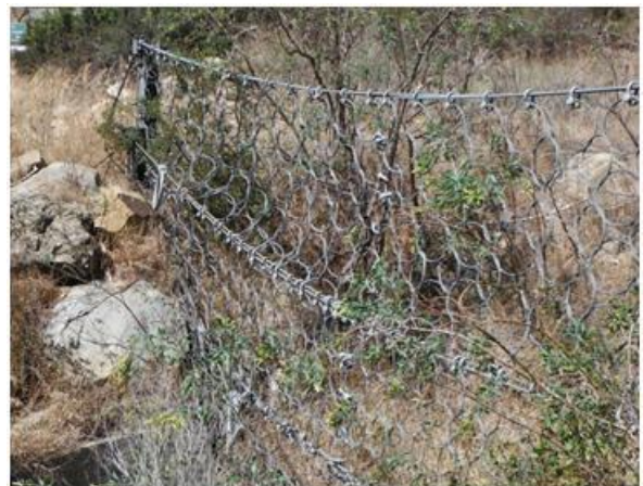
Fig. 16 Flexible type barrier in the channel near the State Highway-1 in California (August, 2013)
