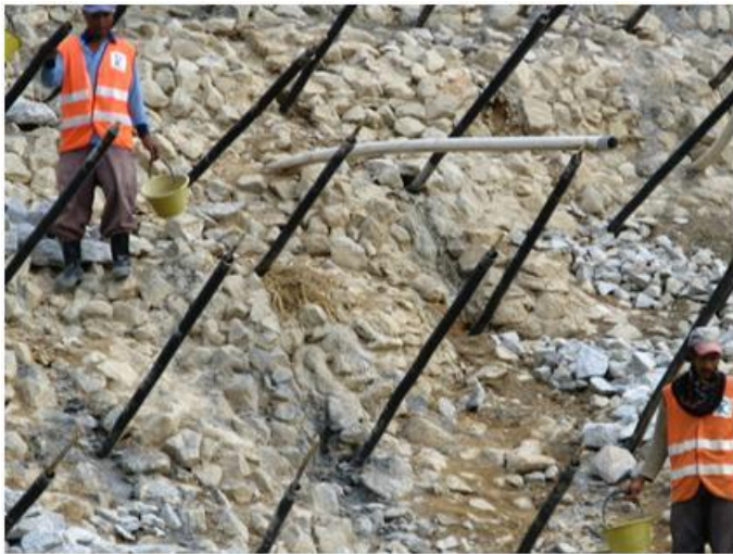
Fig. 20 Photo of the soil nail works along the East-West coast highway from Simpang Pulai to Kuala Berang (May, 2007) .
