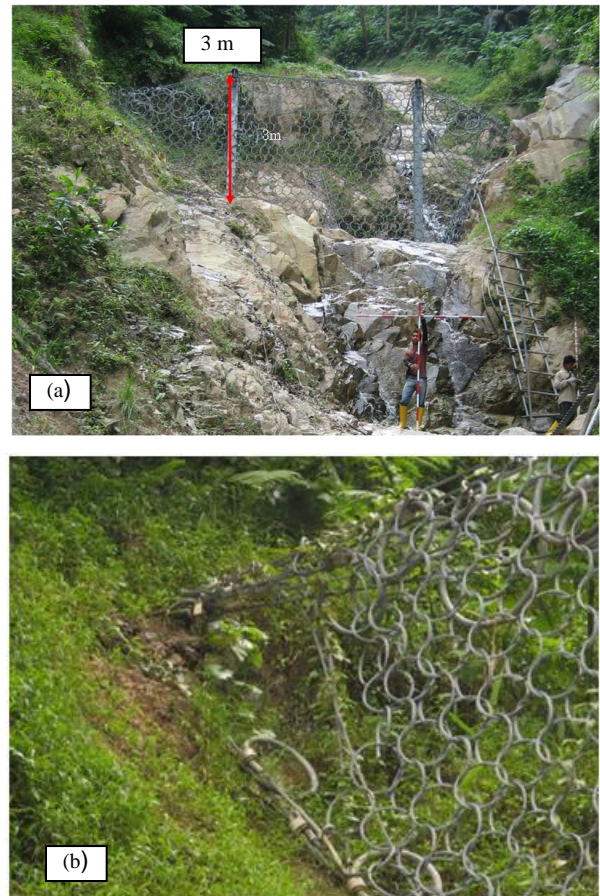
Fig. 15 Three meter high flexible type barrier at Gap Fraser Hill. (a): View from the road; (c) close view of the barrier showing the brakes and the ring net (Ocotober, 2010)
