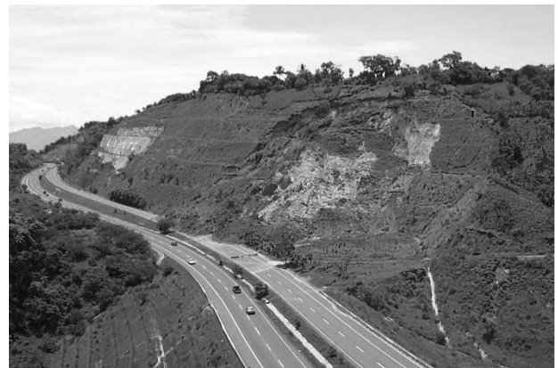
Fig. 25 Bird’s eye photo of the landslide and CA01E taken on January, 2009. (The road is heading towards West).
