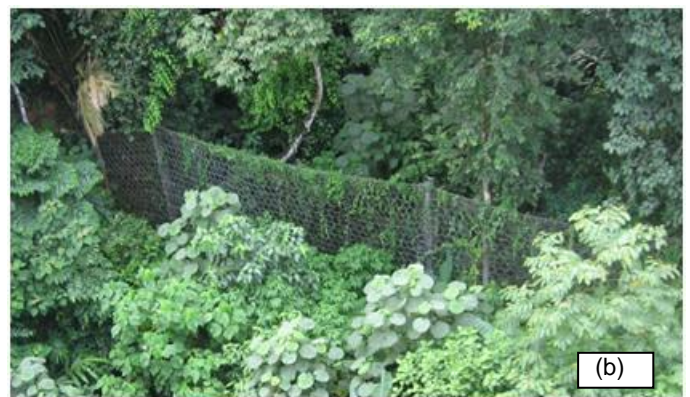
Fig. 13 Flexible type barrier at Gunung Tempurung for capturing debris flow. Photo (a) is taken after the occurrence of debris flow on Ocotober 11, 2004; Photo (b) shows the flexible type barrier in the channel adjacent to the one shown in Fig. 12 (2012, June 28)
