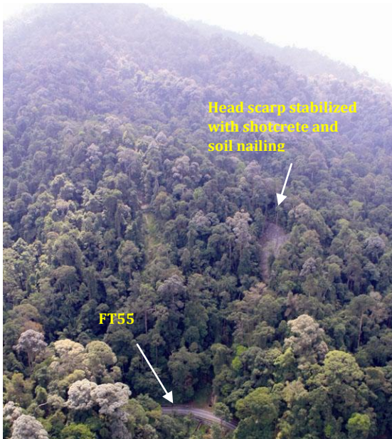
Fig. 17 Aerial photo of the stabilized scarp and the road (FT55) at Kuala Kubu.
