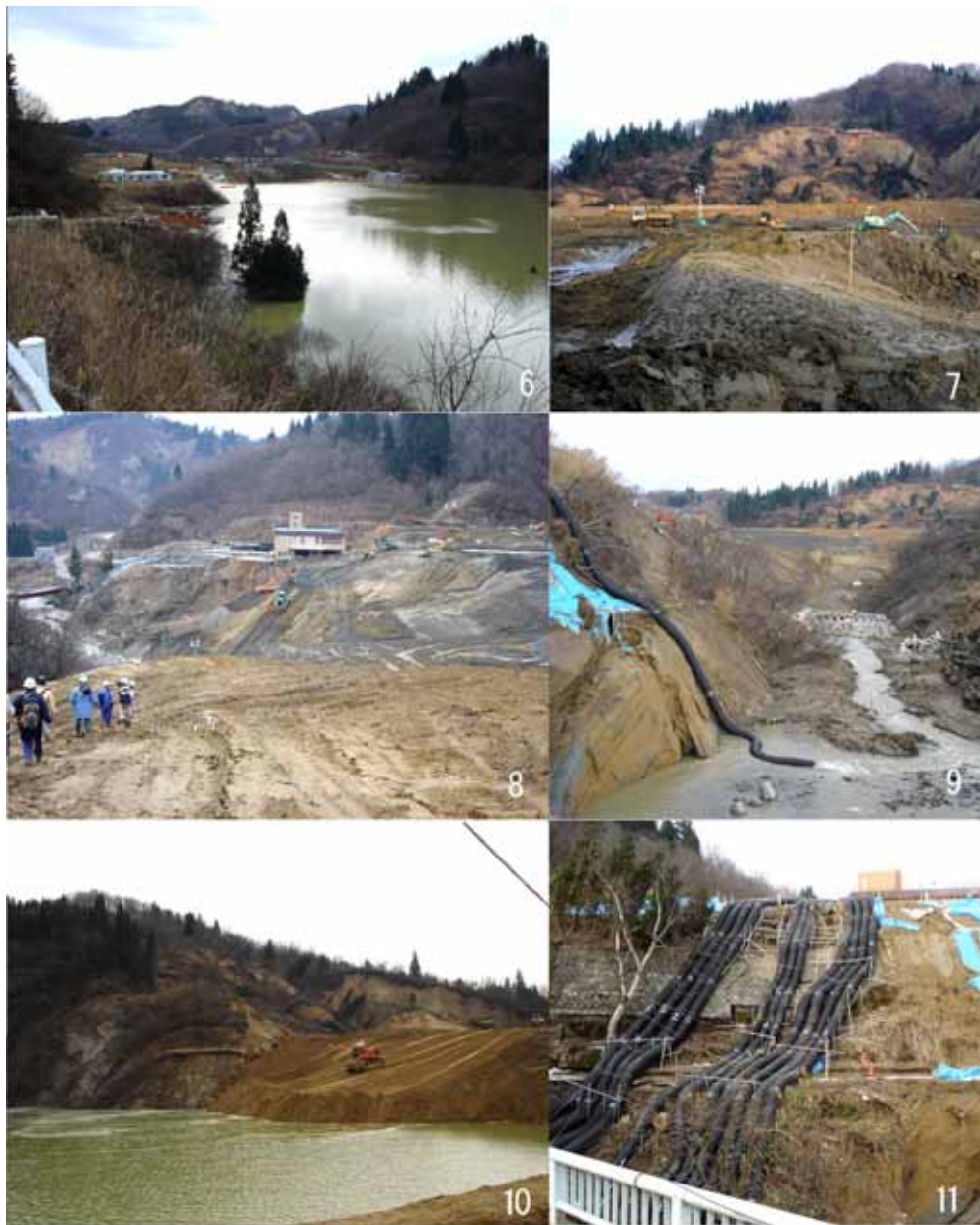
1: Over view of the Higashi Takesawa landslide establishes the large landslide dam at Imogawa river 2: Graben like landform in the landslide body 3: The boundary of the former landslide body and the main scarp 4: Large outcrop of the slip surface 5: Close up the slip surface 6: Landslide dam 7: Repair operation at the surrounding landslides 8: Repairment operation (Cut and fill for the secondary disaster prevention) 9, 10, 11: Cut the canal for water temporal level control
